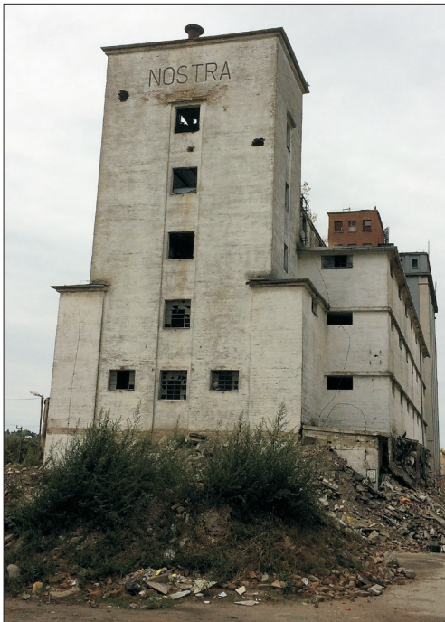
Photo 3. Former industrial building and shelter for homeless people before demolition in Kaposvár
