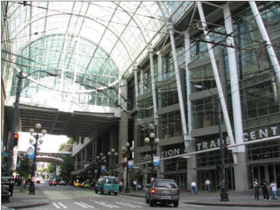
Photo 1. The Washington State Convention Center in downtown Seattle
