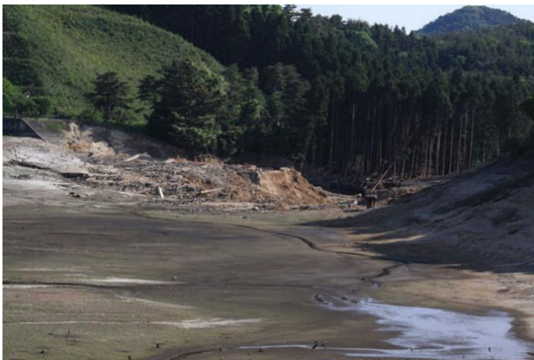
18. ábra. Az összeomlott Fujinuma gát ( https://en.wikipedia.org/wiki/Fujinuma_Dam ) Figure 18. The collapsed Fujinuma dam ( https://en.wikipedia.org/wiki/Fujinuma_Dam )
