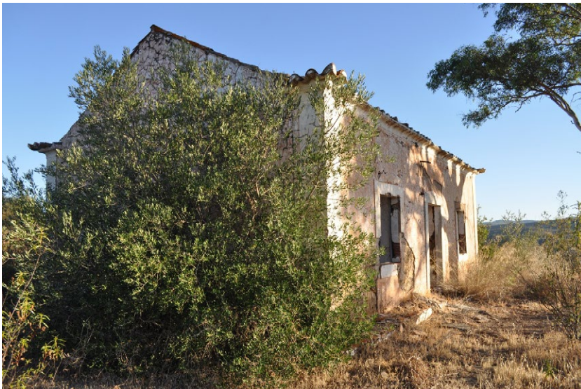
Figure 2: Abandoned Fiscal Guard's house near Alcoutim, Portugal (photo by the author)
